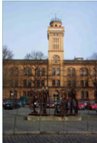
The Physics building of the Martin-Luther-Universität Halle-Wittenberg. The tower was built for astronomical observations, and is still used for that purpose. It also accommodates a Foucault pendulum
